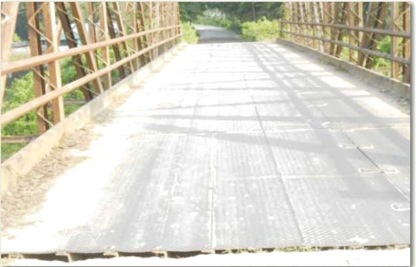
Repair of steel decking on Nonung Nallah
