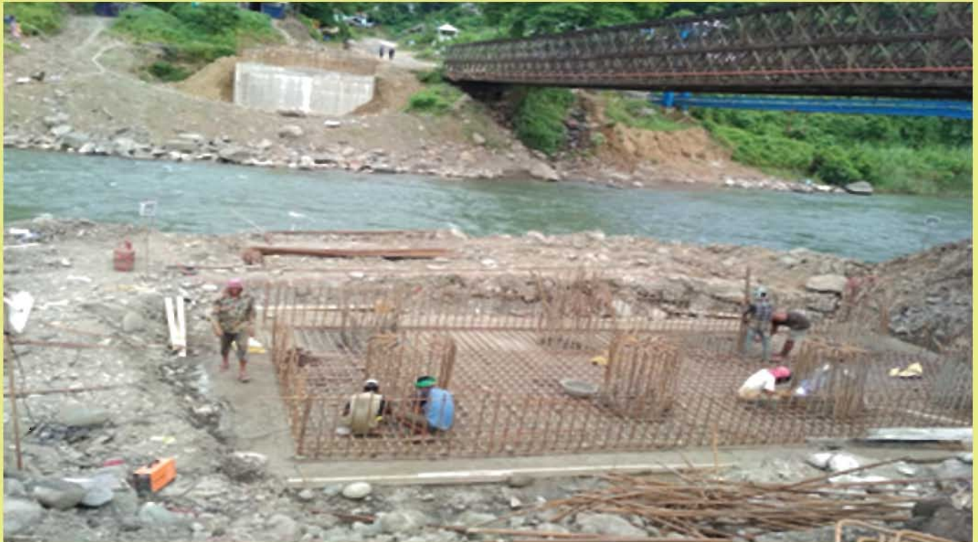
CONSTRUCTION OF SUBSTRUCTURES FOR DOUBLE LANE STEEL COMPOSITE BRIDGE OVER TIRAP RIVER AT CHANGLANG UNDER CRF ( IN PROGRESS ) SH : ABUTMENT SHAFT
