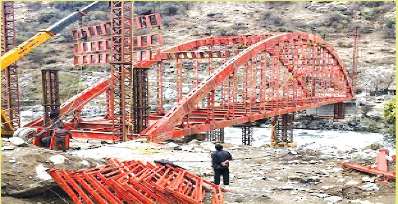
CONSTRUCTION OF STEEL ARCH BRIDGE (60.00 M SPAN) ON ROAD FROM MURGA BRIDGE TO RHO VILLAGE UNDER NLCPR
