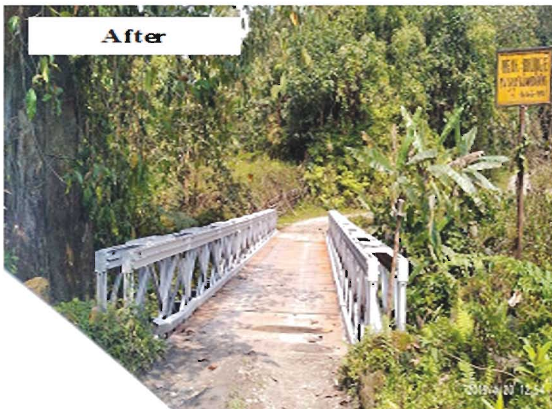
Repair and maintenance of Bailey Bridge on Pasighat-Ledum Tene Koyu road
