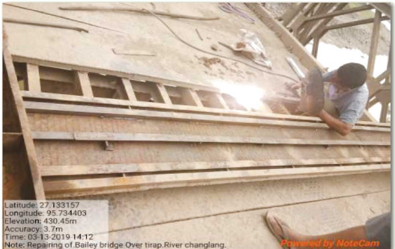
Repairs of cross bracings of Bailey bridge over Tirap river at Changlang
