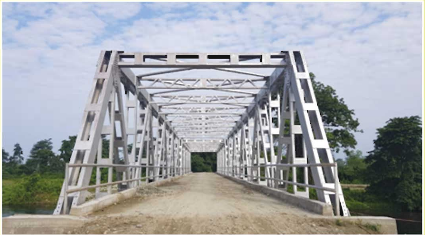
STEEL BRIDGE OVER TIYANG RIVER ON ROAD TO MIMEY, NEAR CHOWKHAM UNDER RIDF (SPAN 60.00M)
