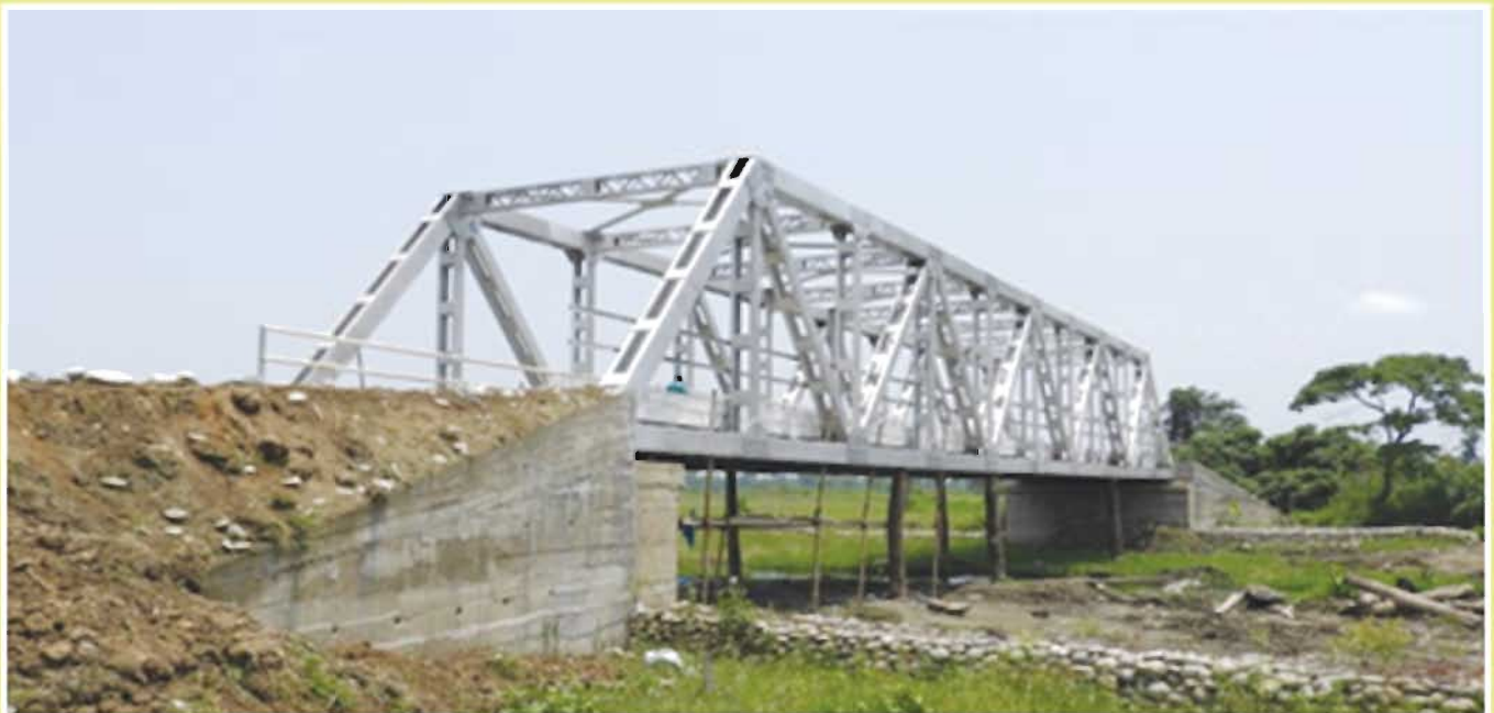
STEEL BRIDGE ON ROAD BETWEEN NEW JENTHU TO JONA III UNDER RIDF (SPAN 40.00M)
