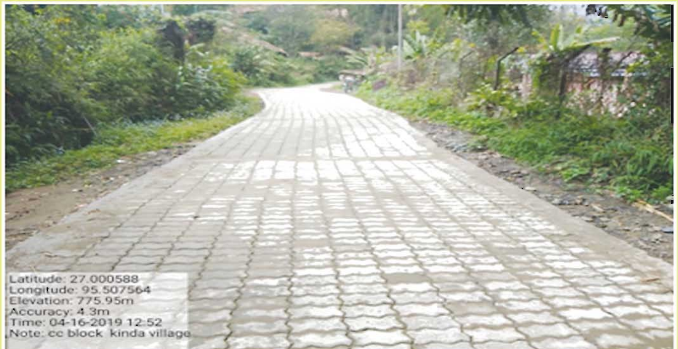
COLONY ROAD NEAR KHONSA TOWNSHIP USING INTERLOCK PAVER BLOCKS
