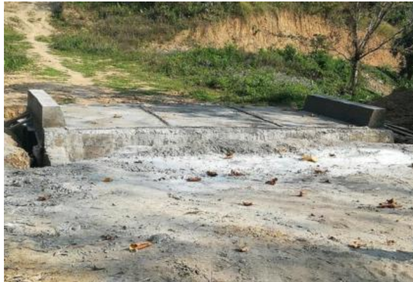
Slab culvert (3m span) at Ch-1.800 Km
