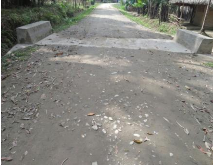
S/Cul-1m span at Ch. 0.015 Km
