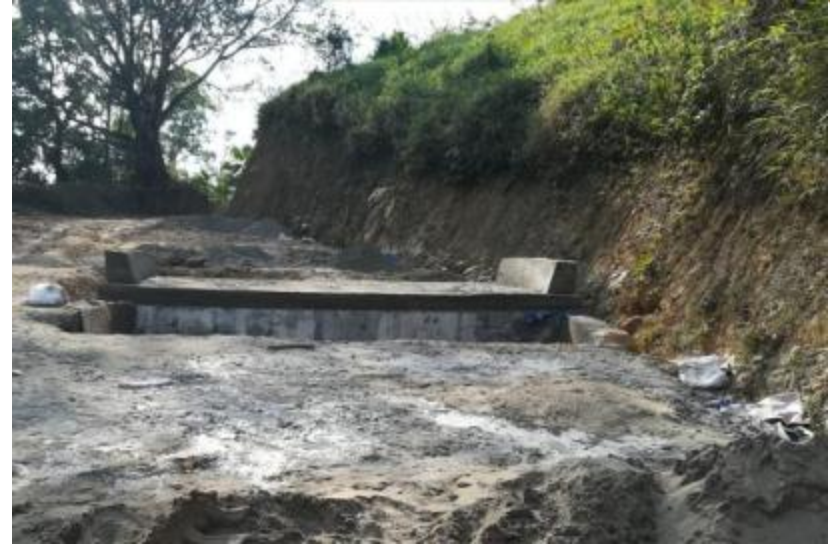
Slab Culvert (2m span) Ch-1.580 Km
