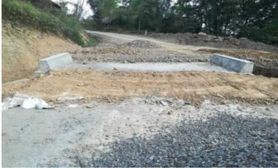
Slab culvert (2m span) at Ch-3.580 Km
