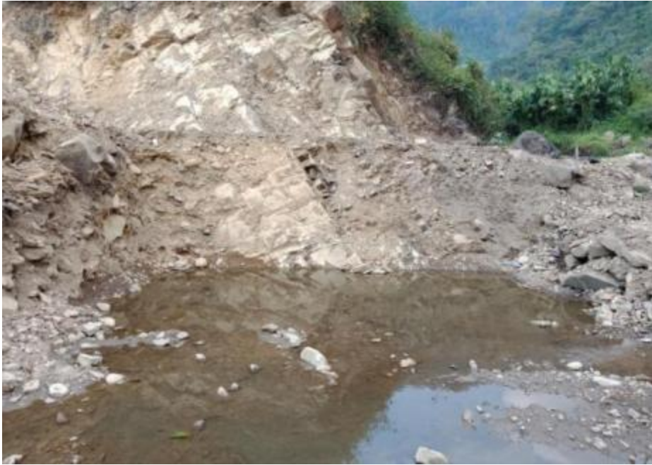
Foundation 25mtr span RCC Bridge at Ch-4.060 Km
