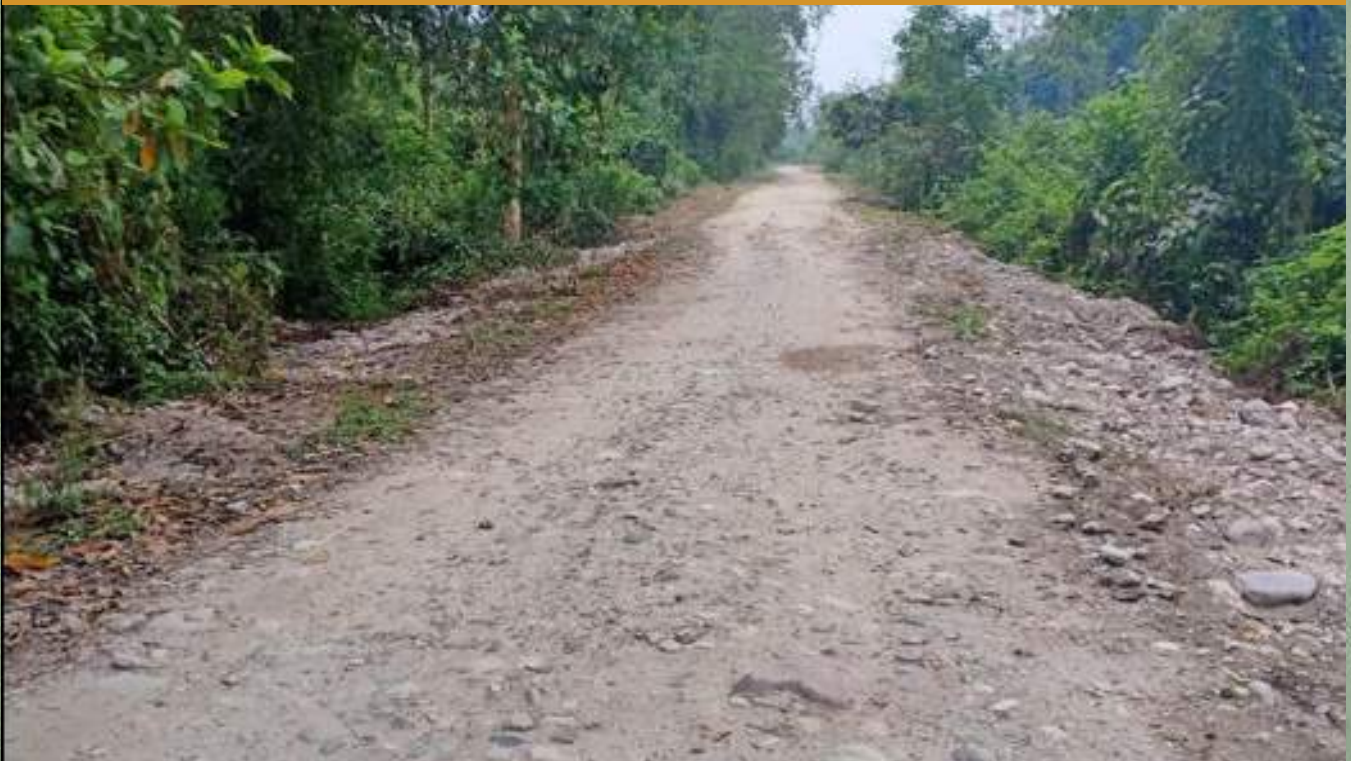
Jungle and Berm Clearance and repairs of WBM surface
