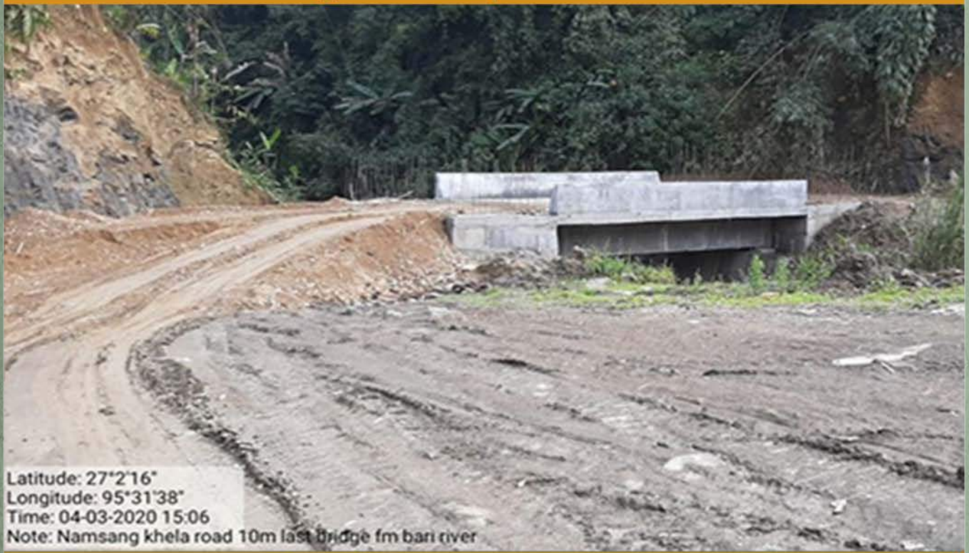
Construction of Namsang Khela Road (21 Km) RCC Bridge 10 mtr Span at Ch 42.37 Km
