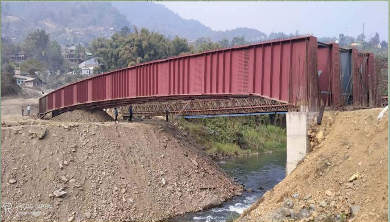
Composite Steel Bridge (Span 60 mtr) over Tirap River in Changlang Town (in progress)(Steel Girders Erected)
