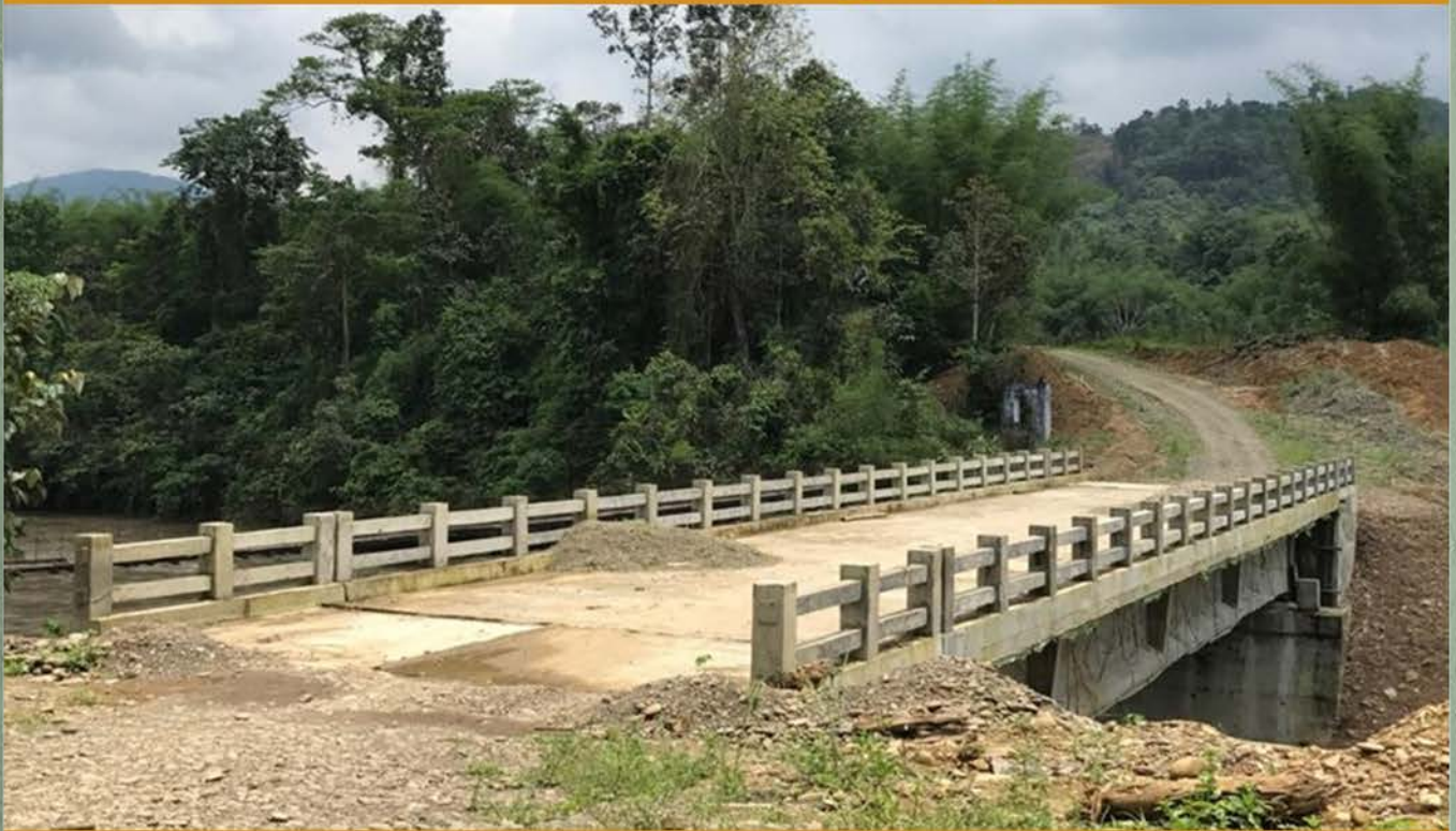
RCC Bridge (Span 30 mtr) over Namchik River to connect Hetlong village
