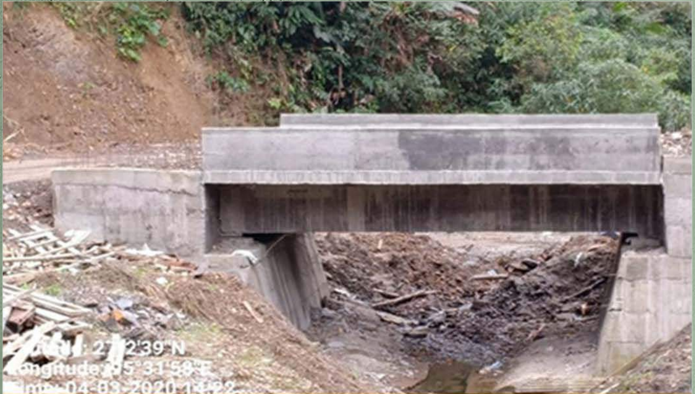
Construction of Namsang Khela Road (21 Km) RCC Bridge 10 mtr Span at Ch 39.49 Km
