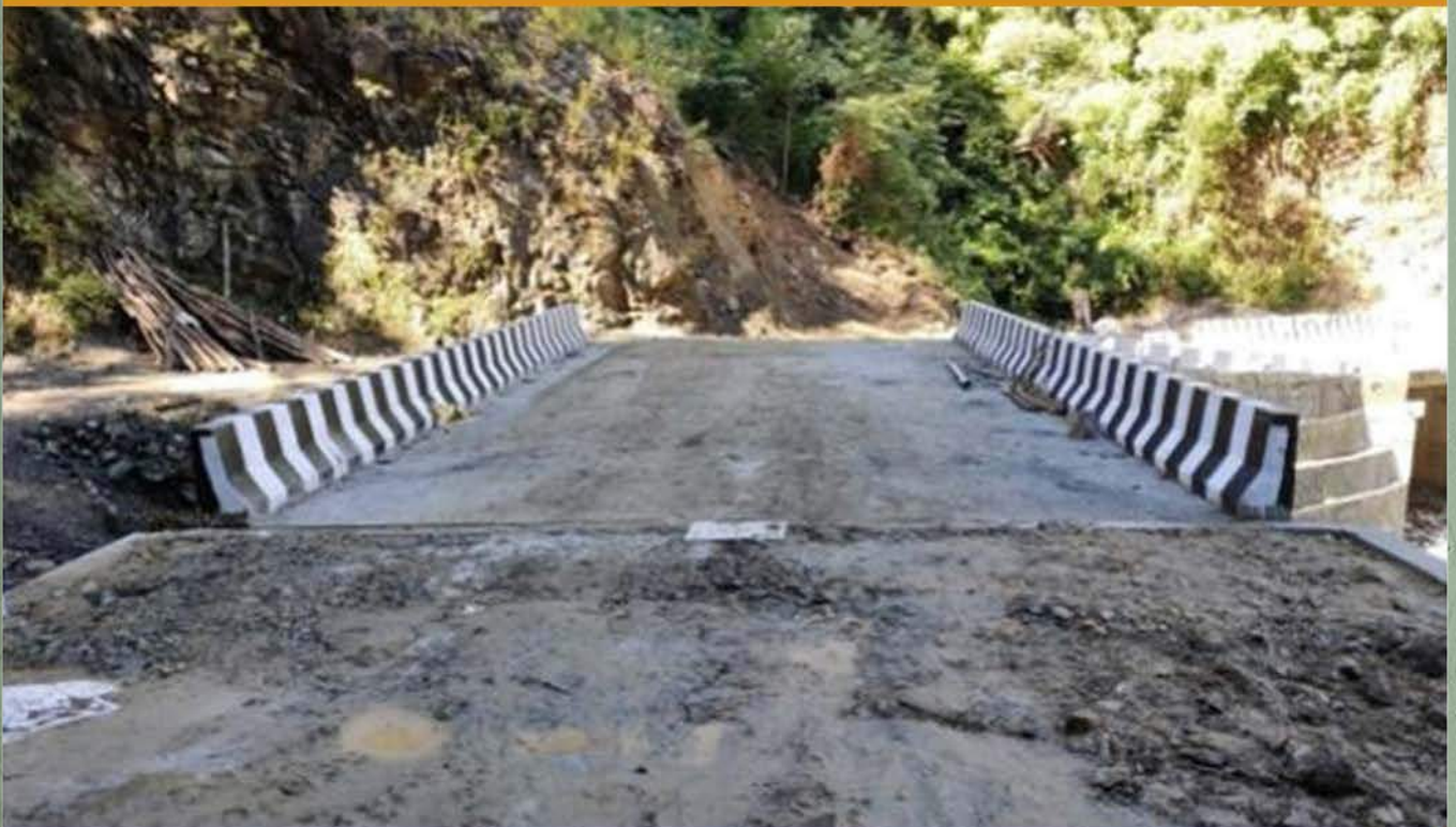
Construction of Bridges on Road from Hawaii District HQ to Manchal Admn Circle(PH-II)RCC Bridge at Ch-13.54 Km(Span - 10 mtr)
