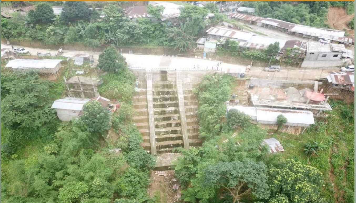
C/o Protection wall and culvert at ESS sector, Itanagar
