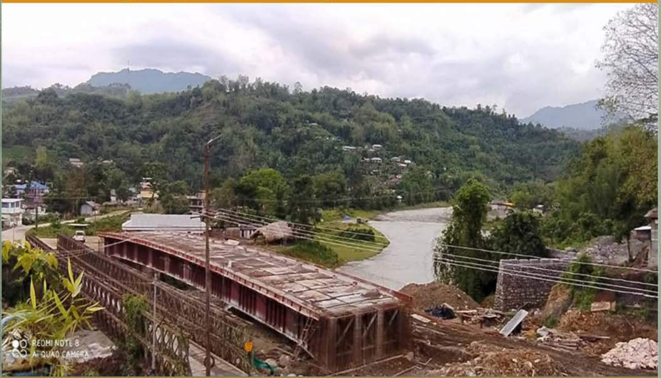
Composite Steel Bridge (Span 60 mtr) over Tirap River in Changlang Town (in progress)(Deck Slab Concreting completed)
