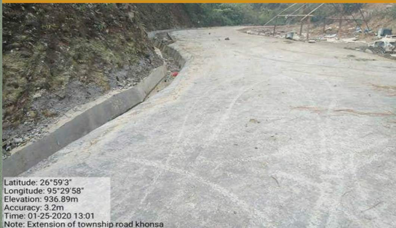
Extension of Khonsa Township Road Cement Concrete Pavement with Side Drains at Ch 0.880 Km
