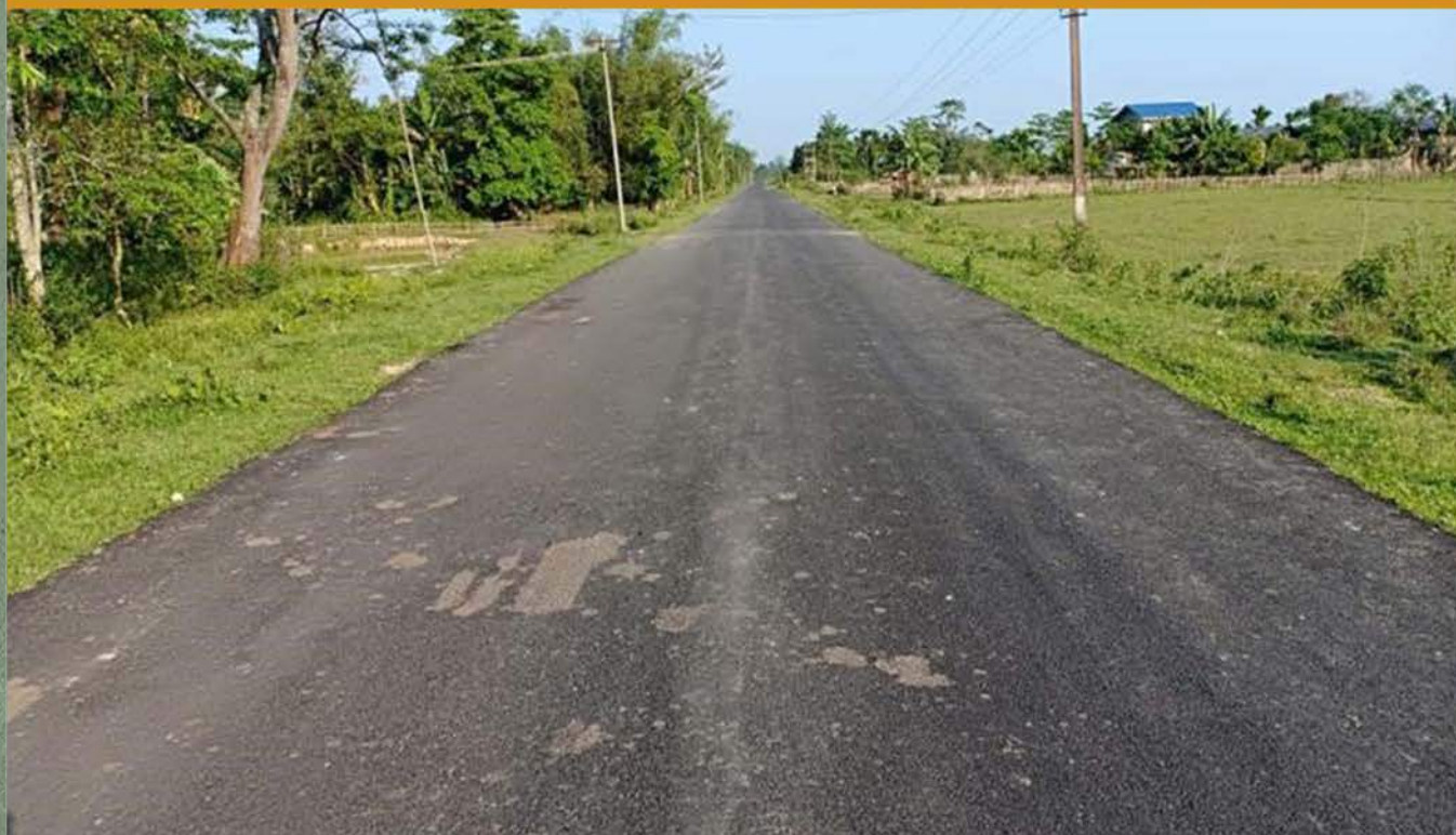
Construction of various roads and bridges under Lekang circle, Namsai Carpetting 5.50m width at Chainage 7.50 Km
