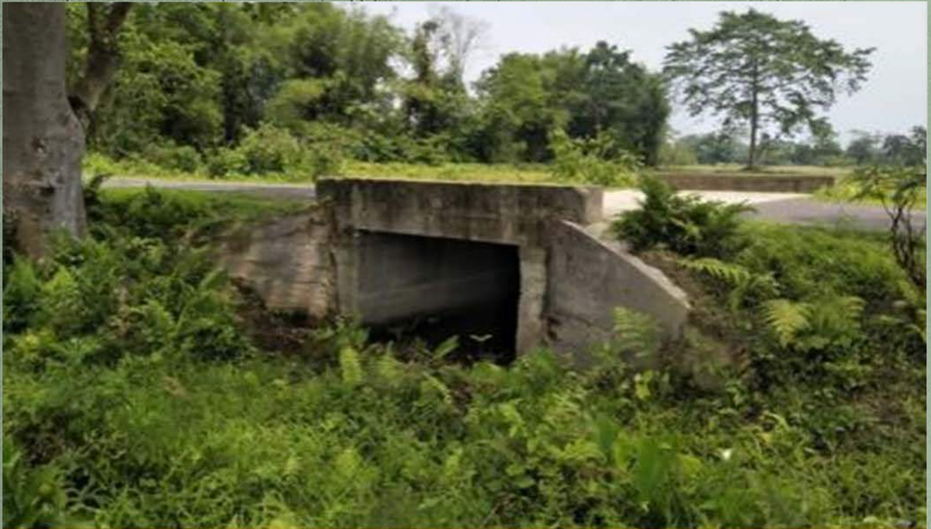
Construction of road from Nongsaya village to Menkengmiri in Namsai District RCC Slab Culvert 2.00 Mtr span-Ch 1.45 KM
