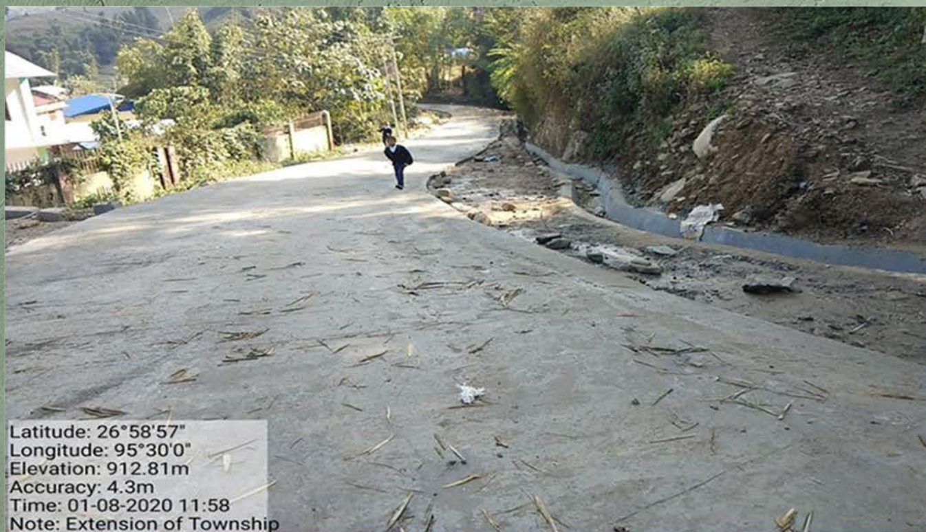
Extension of Khonsa Township Road Cement Concrete Pavement with Side Drains at Ch 1.20 Km
