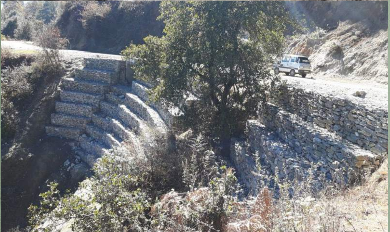
Flood Damage of PWD Infrastructure during recent Flood of 2017-18 under AP (Gabian Structure on Crafrt Centre- Old Lebrang Road)
