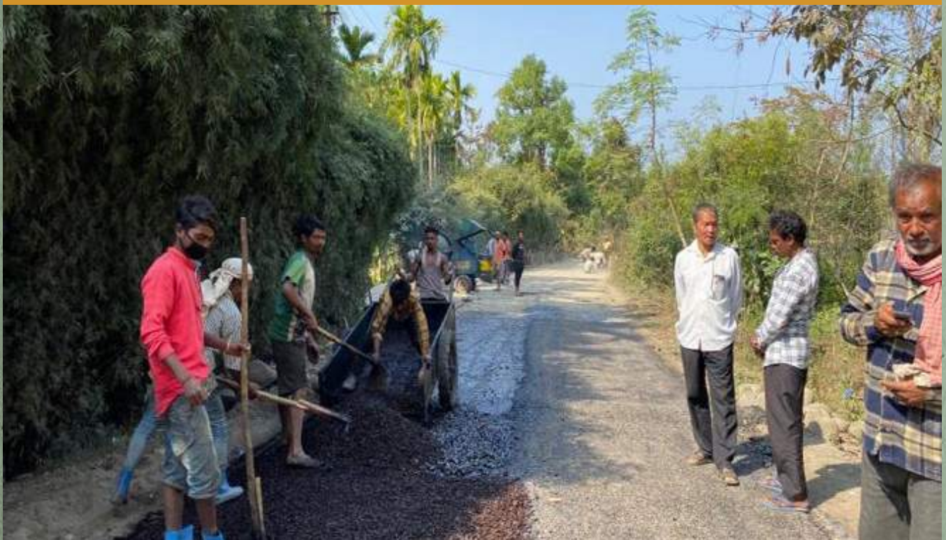
Repairs of potholes and recarpetting of NH 215 to Bordumsa road
