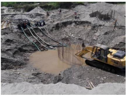
Abutment - Left Bank well sinking in progress
