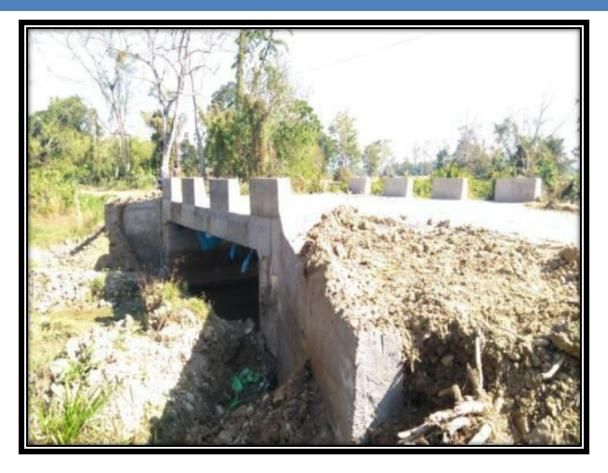
RCC Culvert 6m span at Mokrun Link Road
