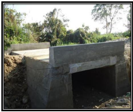
RCC Culvert 1m span at IRBn HQ. Link Road
